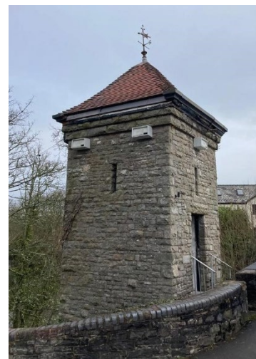
Swift nest boxes installed on the Sennybridge Pumping Station
